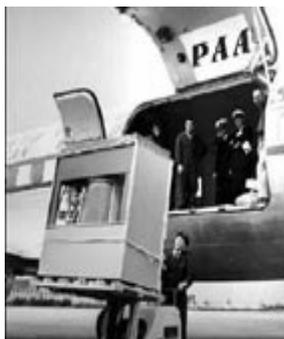
In September 1956, IBM launched the 305 RAMAC, the first computer with a hard drive. The drive weighed over a ton and stored 5 megabytes of data. Makes you appreciate your 4 Gigabyte USB thumb drive, doesn't it?
